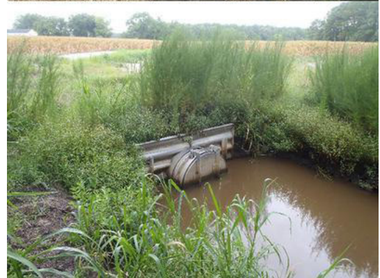
Note: Dike with pump drain attached (top) and floodgates (bottom) in Hyde County. Photo from Carl Crozier.
